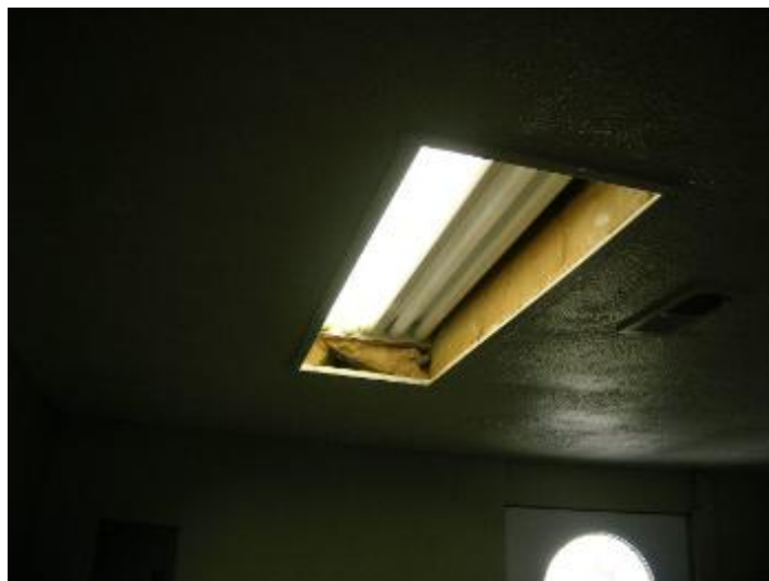
There are missing light covers throughout the house.
