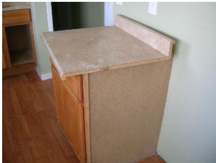
The east counter in the kitchen is not attached to the cabinet.
